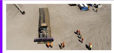
FlexRoad's team sprung into action and traveled to the site, where we deployed the matting and undertook a trial to showcase how strong and versatile it is, even on such unpredictable ground. Taking the weight of heavy shovel loaders and excavators, the matting enabled FBC to access areas necessary to create a trench and drainage plan, and the work continued!
