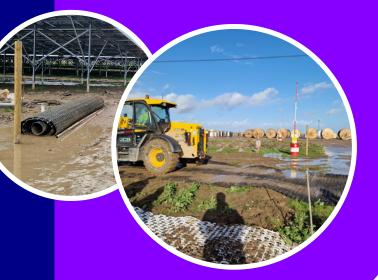
With the project falling behind track, Mytilineos needed a reliable and effective solution, and approached FlexRoad for help. FlexRoad's team was quickly on hand to supply and deploy matting for main access roads, enabling workers and vehicles to move about the site with ease.
